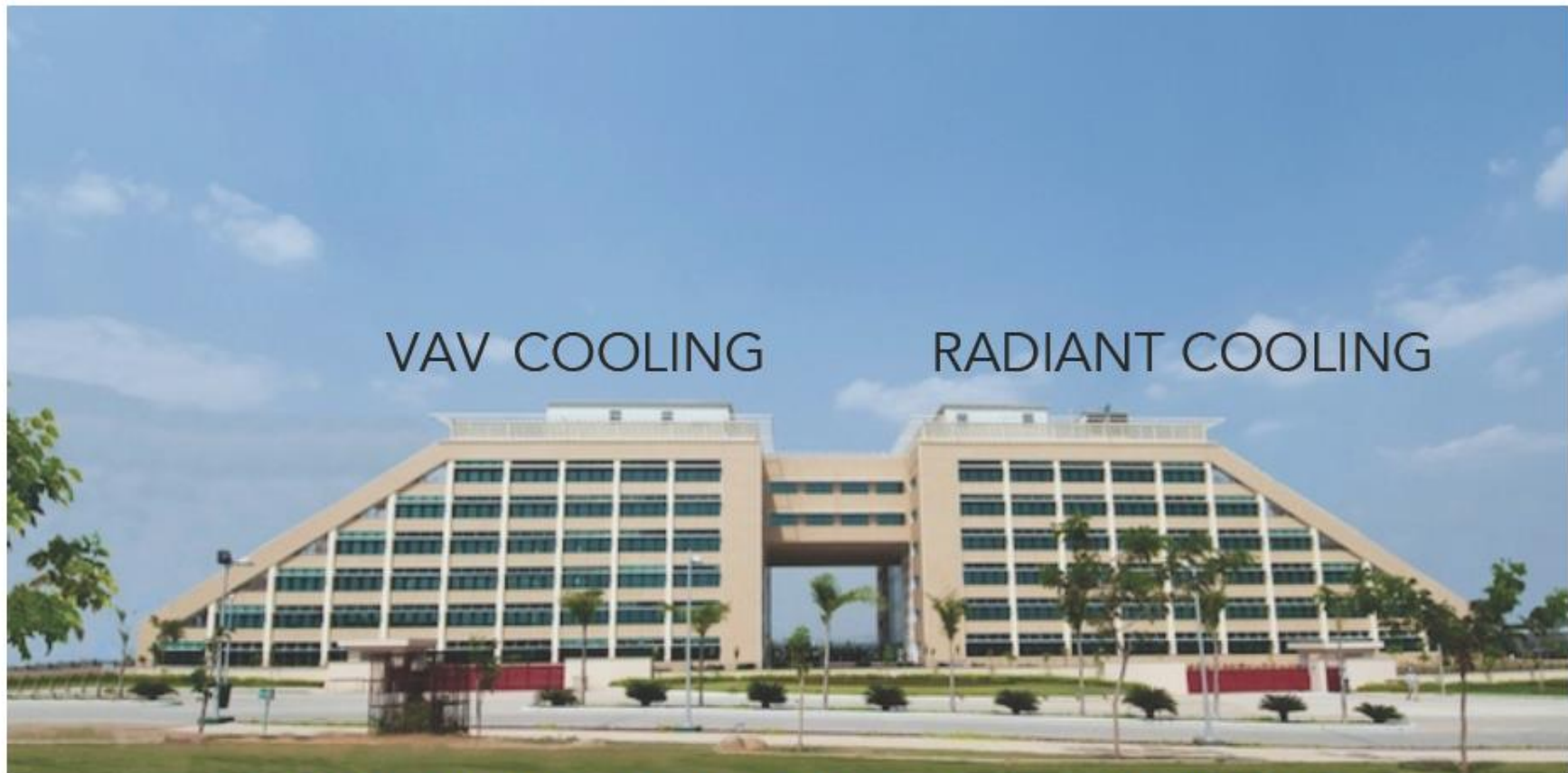
Figure 1 - Infosys SDB-1 Hyderabad - 125,000 sf of radiant cooling and 125,000 sf of VAV cooling
