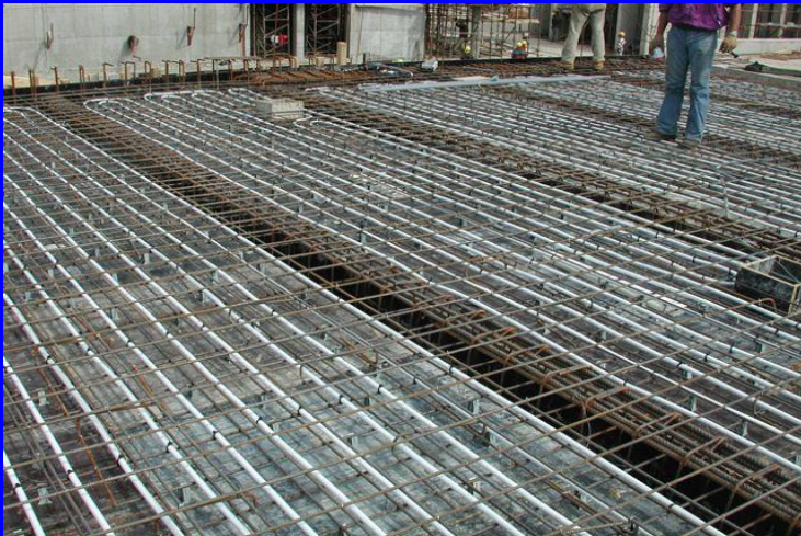
Pipe installation: American University in Beirut, Lebanon Fixing of Uponor MLCP to steel-mesh which will then be covered by concrete
