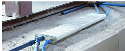
Figure 4. Alternative solution of recovery of waste heat using a heat exchanger placed under the shower tray. SV1 = squared shower tray with drain, in the middle, RP2 = heat exchanger - regenerative panel placed under the shower tray, S = wall-mounted thermostatic shower mixer.
